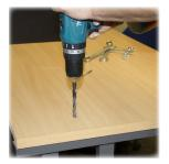
When drilling ensure the drill is kept straight to avoid the screen sitting out of line.
